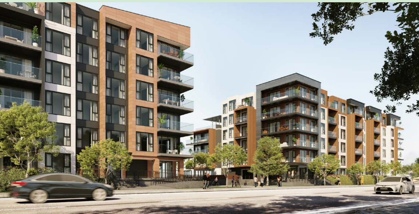
CREDIT: Ignite Architects
